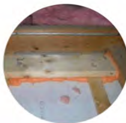
Gaps 1/4 " – 3" Spray foam
