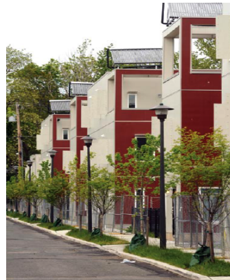
In the fall of 2011, Asociación Puertorriqueños en Marcha completed 13 new LEED Gold homes that use solar hot water systems to help residents reduce the cost of hot water.
